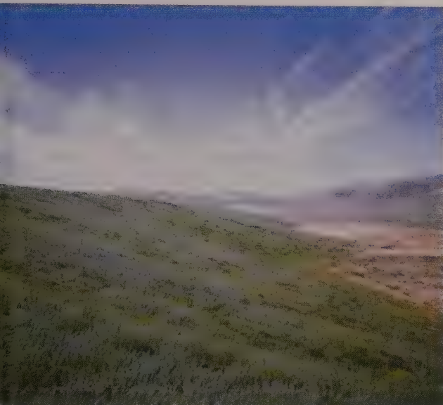
This reclaimed waste rock pile, at the Marigold Mine in Nevada, has been recontoured, covered with topsoil, and seeded with grass.
